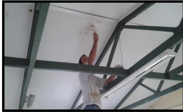
Michael - Sealing the water leaks on the ceiling
